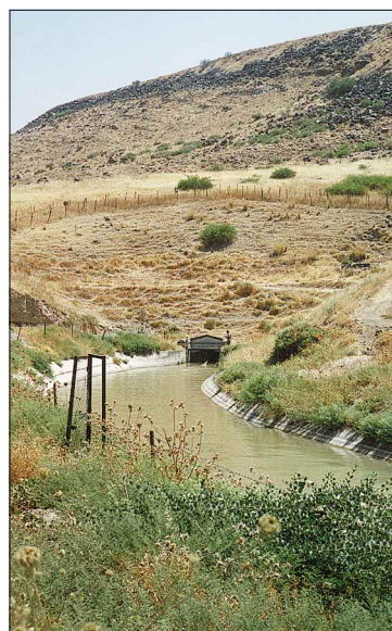
Water distribution systems, such as the Israeli National Water Carrier and the Jordanian King Abdullah Canal, distribute water from areas of water surplus to areas of water deficiency. The northern end of the King Abdullah Canal, shown here, receives water diverted from the Yarmouk River via a 900-meter (m) long tunnel.
